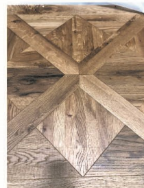
COLOUR VARIATION/ MEDULLARY RAYS/SAW MARKINGS
