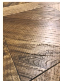
SPLITS IN TIMBER/ SAW MARKINGS
